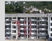
Delta Sunshine Teaching Building, Dazhai High School, Yunan First prize project replication of Delta-Cup International Solar Building Design Competition
