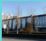
Beijing Office LEED Silver
