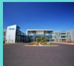
Americas HQs LEED Platinum WELL HSR
