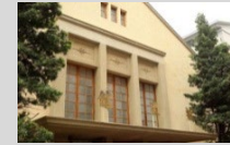
Historical Lecture Hall, Taichung First Senior High School Restoration in Green Building concept
