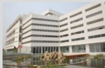
NCKU Delta Building EEWHDiamond
